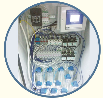
Reactive strength compensation cabinet for street lighting networks
