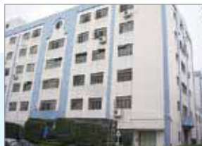
MEAN WELL GUANGZHOU TIANHE R&D CENTER
