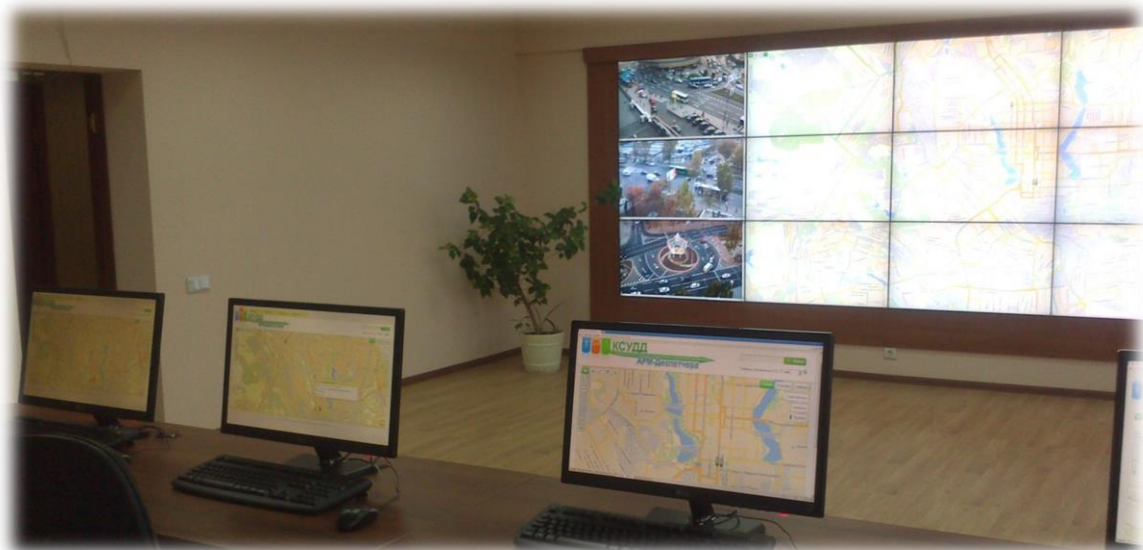
Integrated Traffic Management Systems
