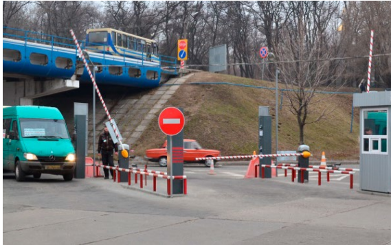
Parking complexes for bus and railway stations
